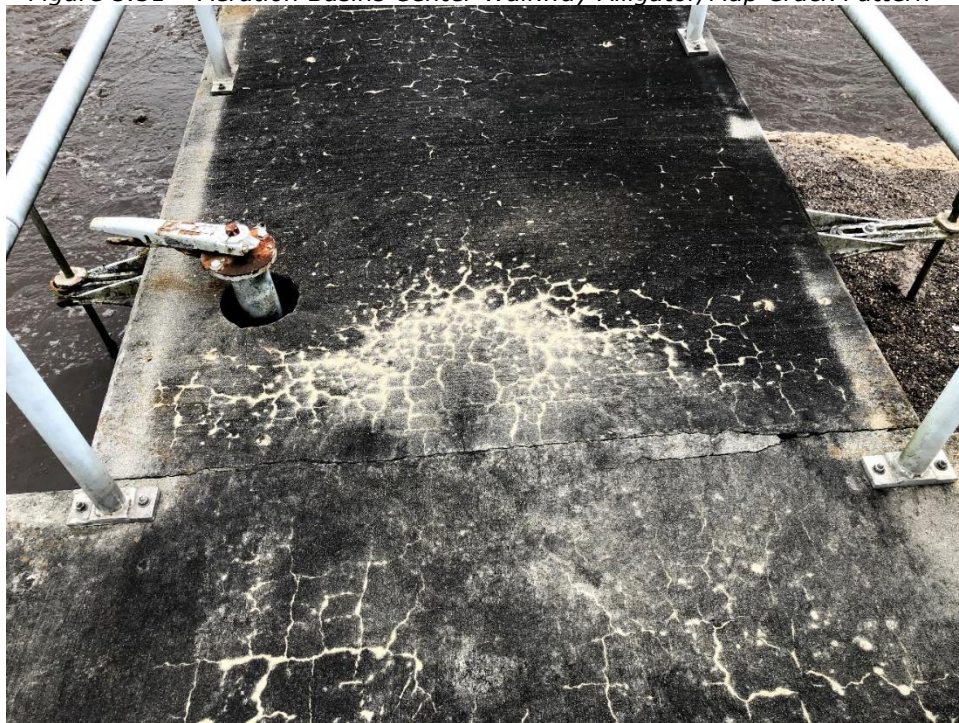
Figure 5.51 – Aeration Basins Center Walkway Alligator/Map Crack Pattern
