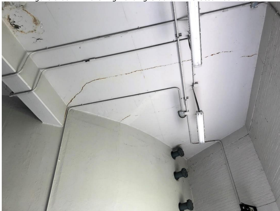
Figure 5.88 – Thickening Building Cracks in Elevated Roof Slab
