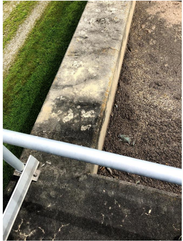
Figure 5.51 – Aeration Basins Center Walkway Alligator/Map Crack Pattern
