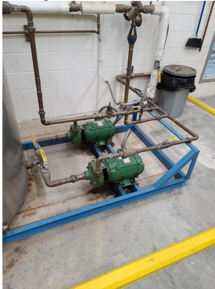
Figure 5.74 – Plant Seal Water System
