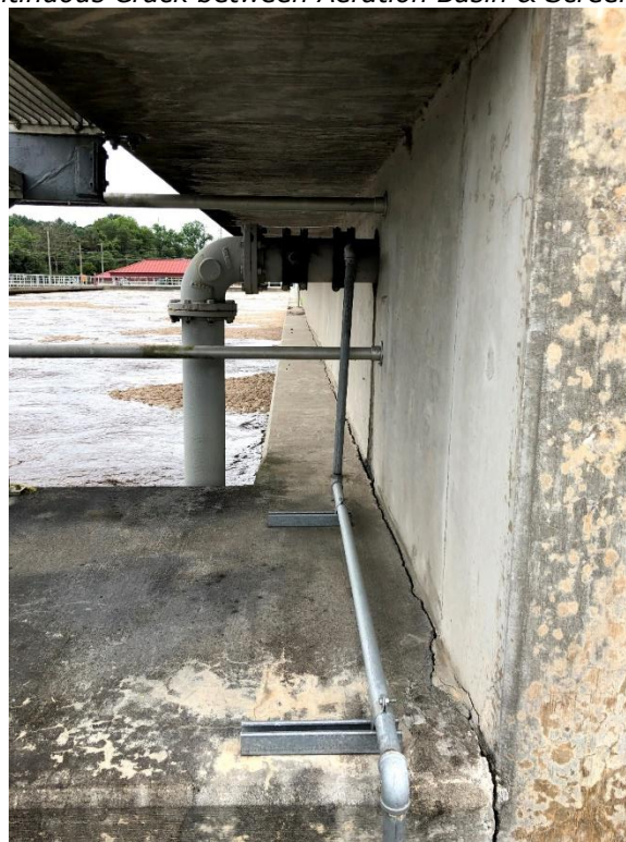
Figure 5.42 – Continuous Crack between Aeration Basin & Screening/Grit Removal
