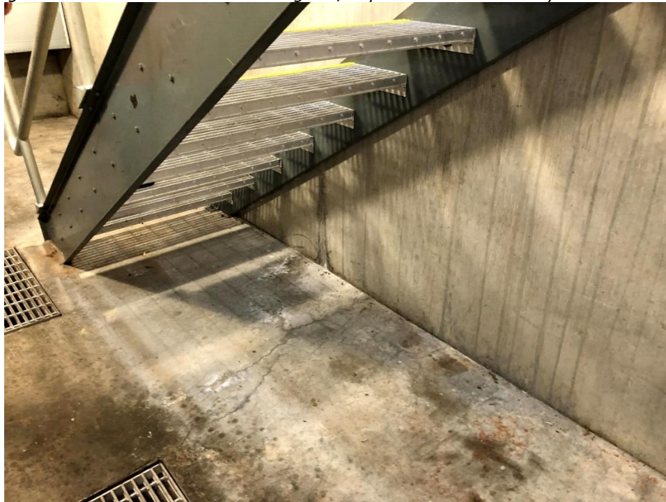
Figure 5.67 – Linear Cracks and Alligator/Map Crack Pattern in Dry Pit Floor Slab
