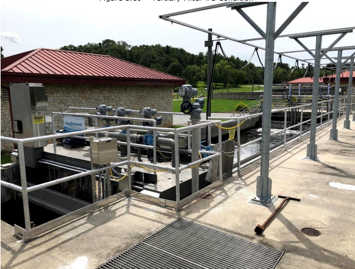
Figure 5.69 – Tertiary Filter #1 Condition
