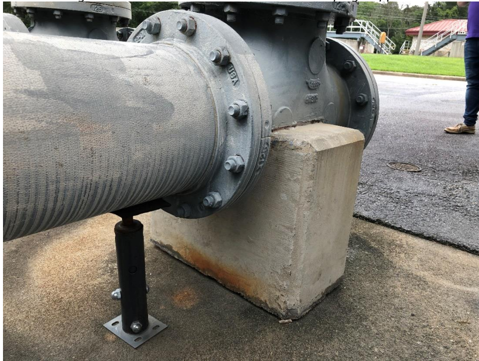
Figure 5.103 – Slab Settlement at Blower Piping Support
