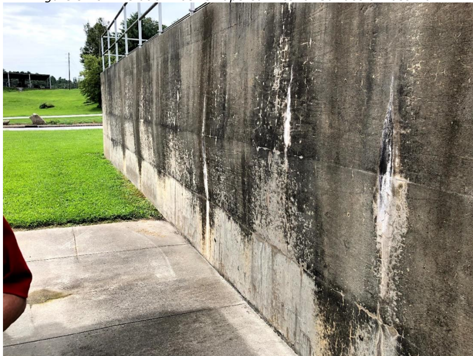
Figure 5.48 – Aeration Basins Tapered Exterior Surface of East Wall
