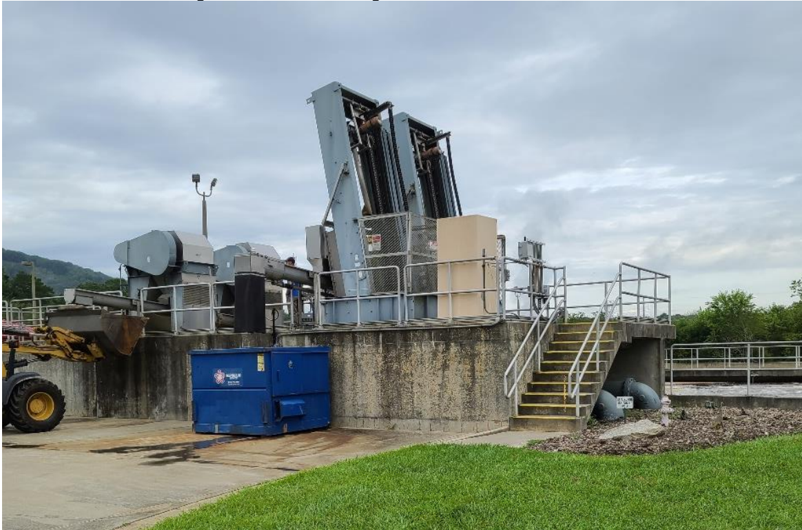
Figure 5.38 – Screening and Grit Removal Structure
