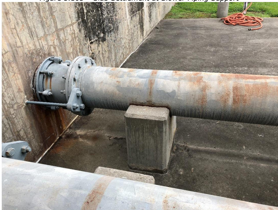
Figure 5.103 – Slab Settlement at Blower Piping Support
