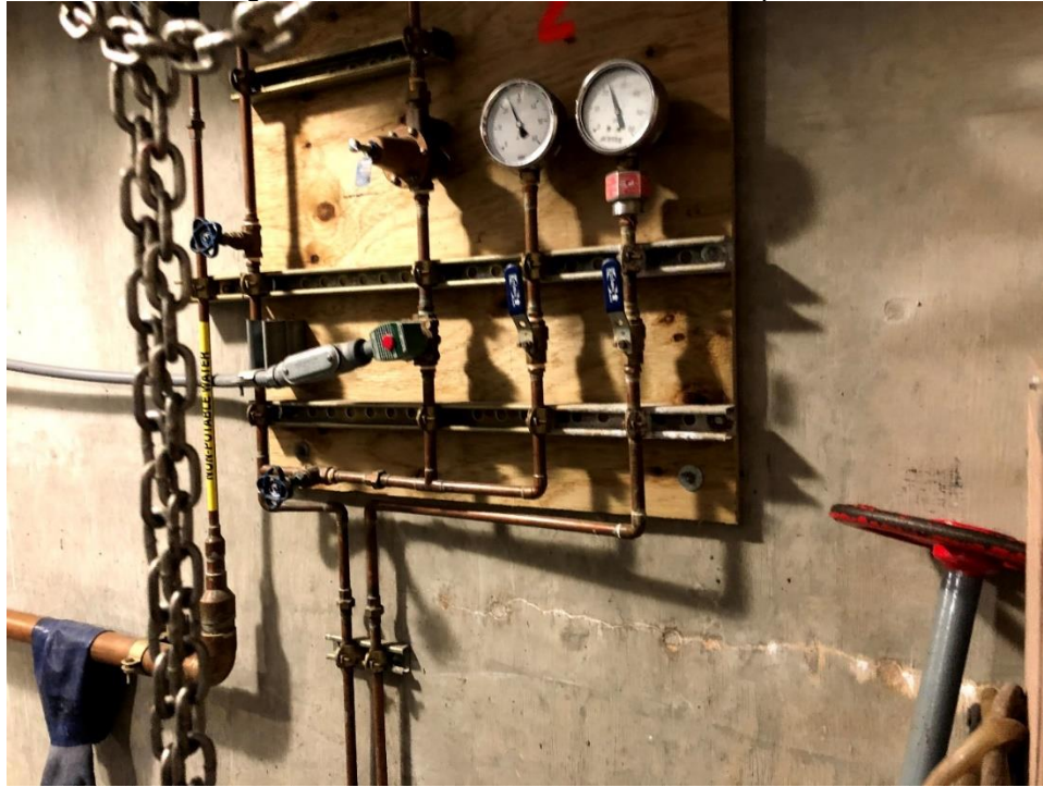
Figure 5.64 – RPS Horizontal Crack in Dry Pit
