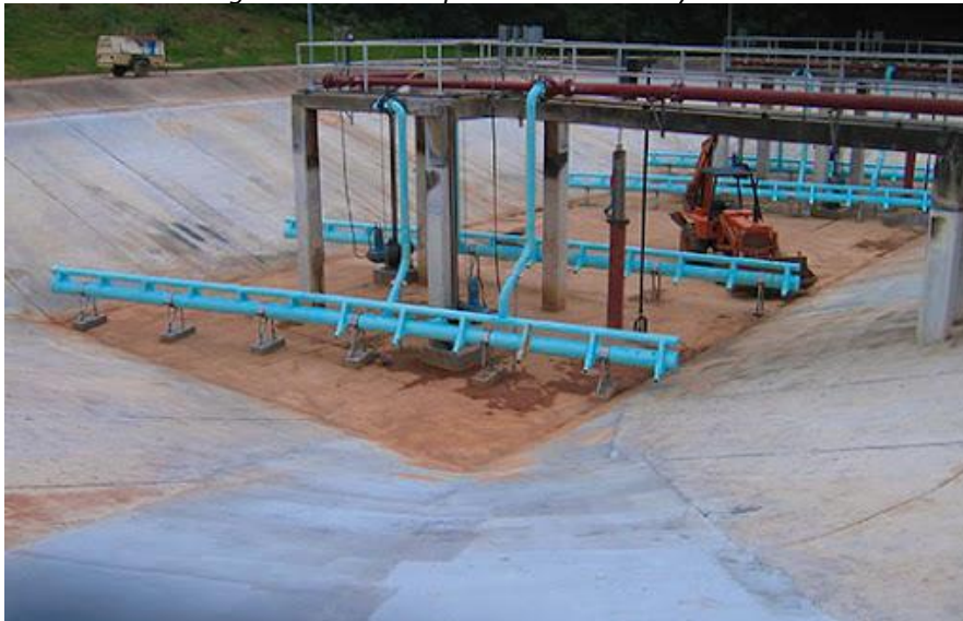
Figure 6.2 - Example Jet Aeration System
