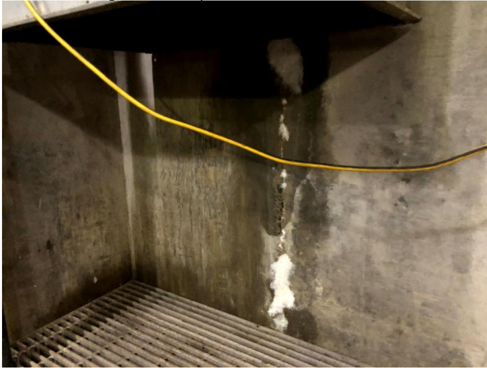
Figure 5.31 – Large Crack at Top of Wet Well Wall
