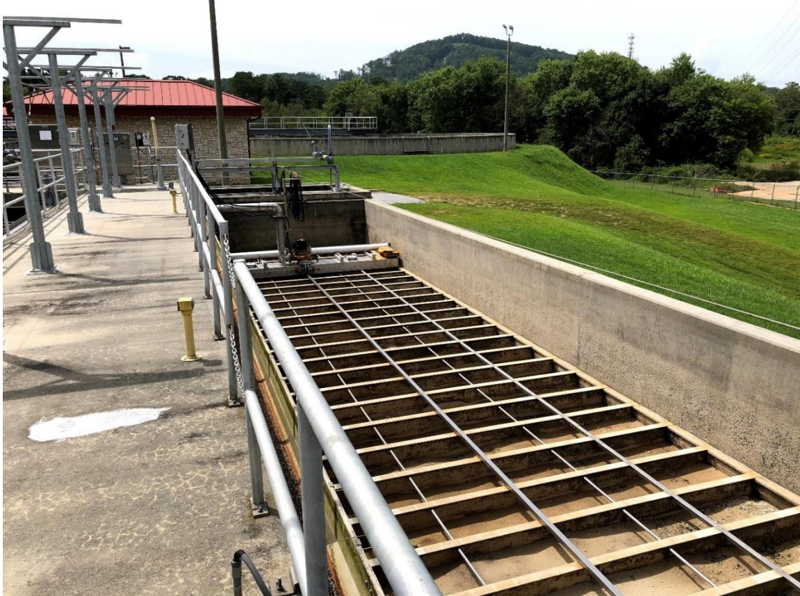
Figure 5.68 – Tertiary Filter #2 Condition
