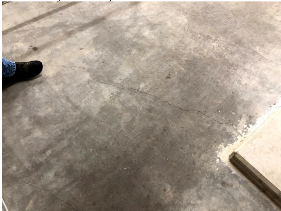
Figure 5.35 – Dry Pit Cracks in Elevated Floor Slab
