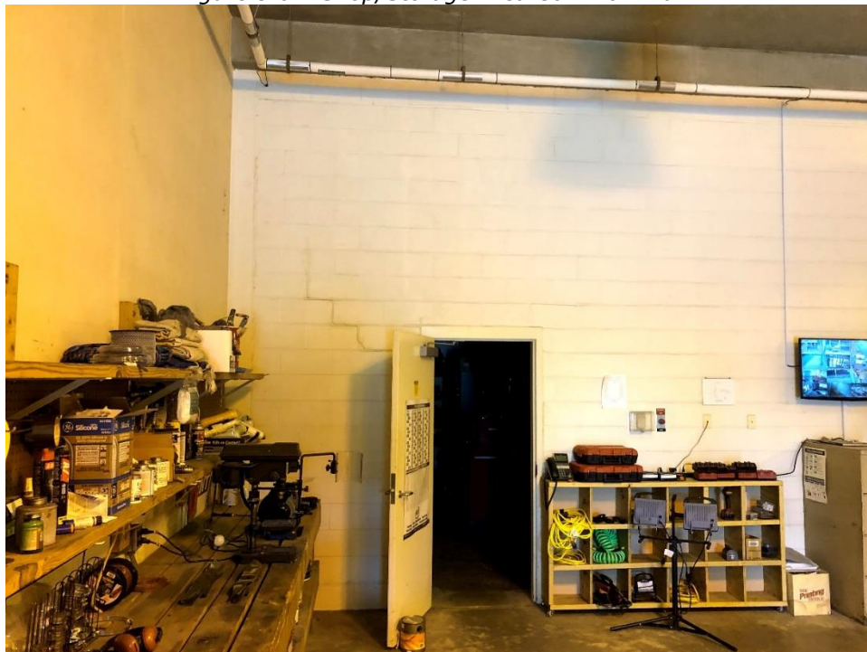
Figure 5.6 – Shop/Storage Area Common Wall
