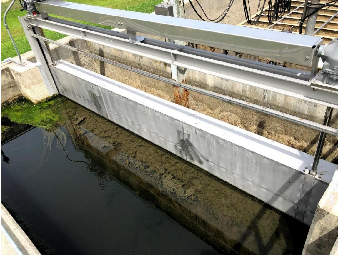
Figure 5.70 – Filamentous Algae growth in Tertiary Filter Influent Channel
