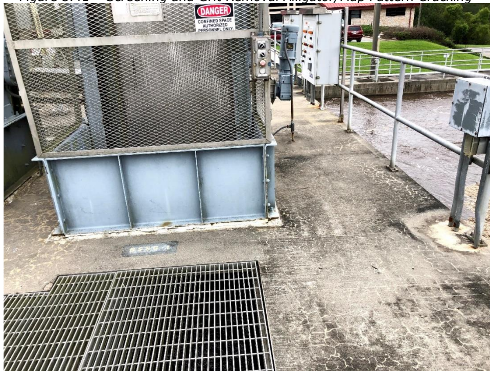
Figure 5.42 – Continuous Crack between Aeration Basin & Screening/Grit Removal
