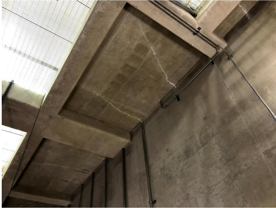
Figure 5.35 – Dry Pit Cracks in Elevated Floor Slab
