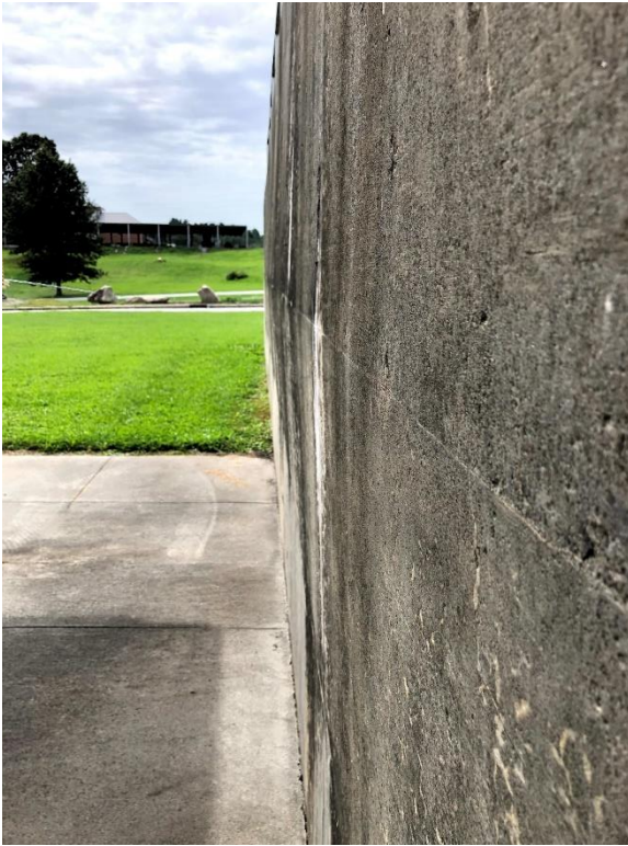
Figure 5.51 – Aeration Basins Center Walkway Alligator/Map Crack Pattern
