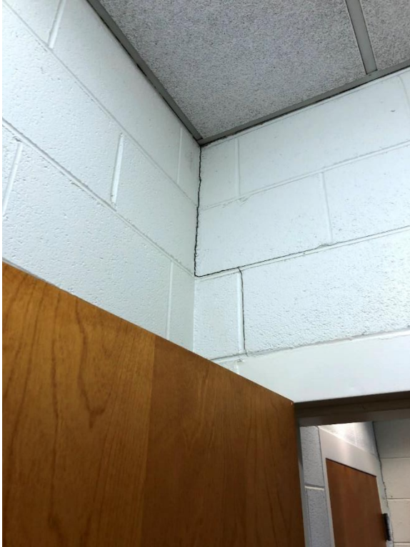
Figure 5.11 – Laboratory Office Cracks in CMU Wall
