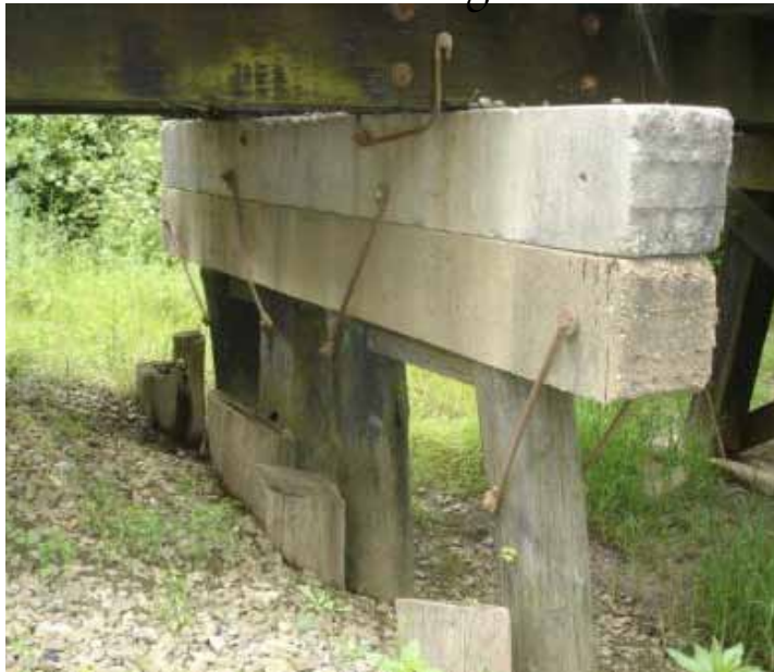
Typical Bent Section
