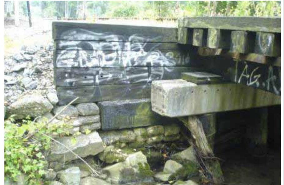
Tie and Timber Deterioration
