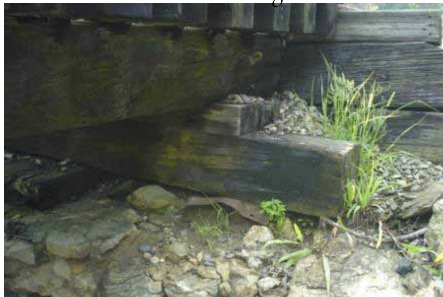
North Back Wall Undermining
