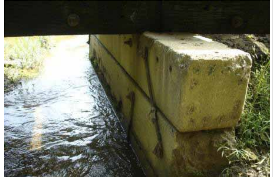
South Back Wall
