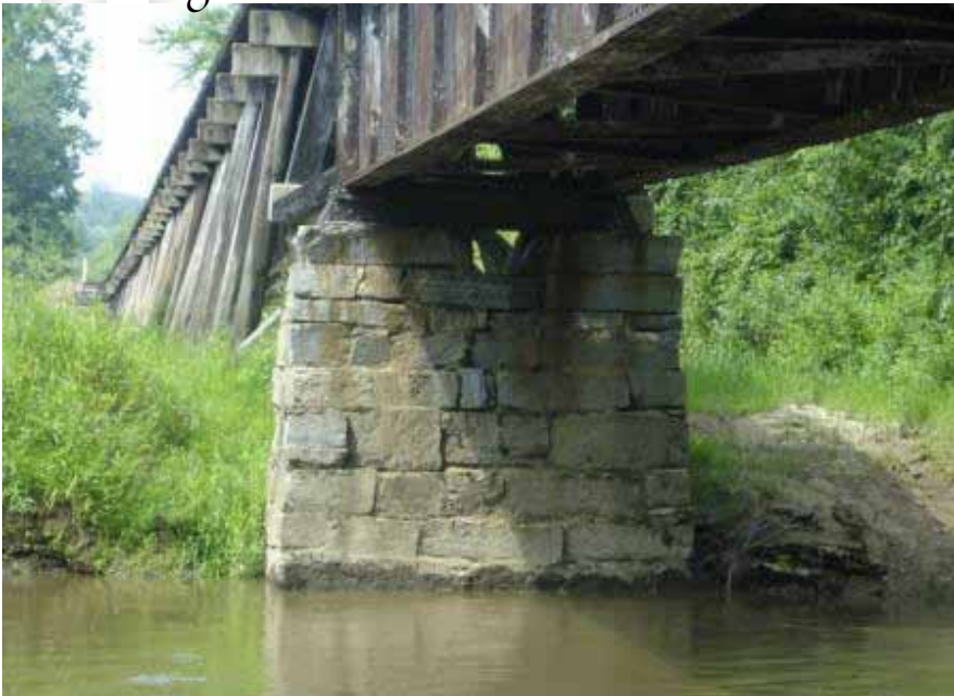
Steel Bridge Foundation
