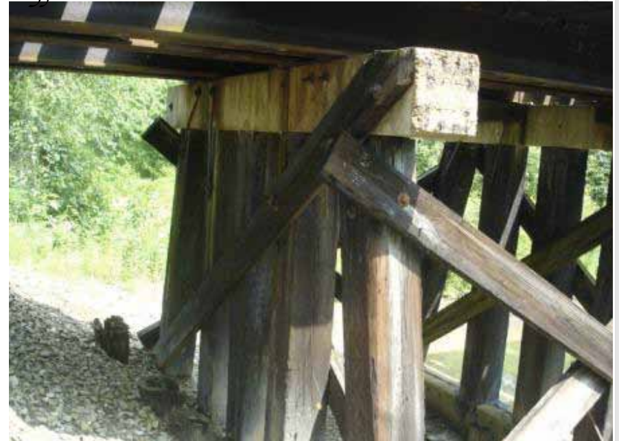
Bent Foundation Undermining
