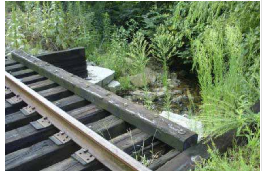
Tie and Timber Deterioration
