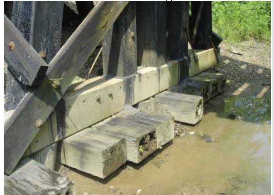
Bent Foundation Undermining
