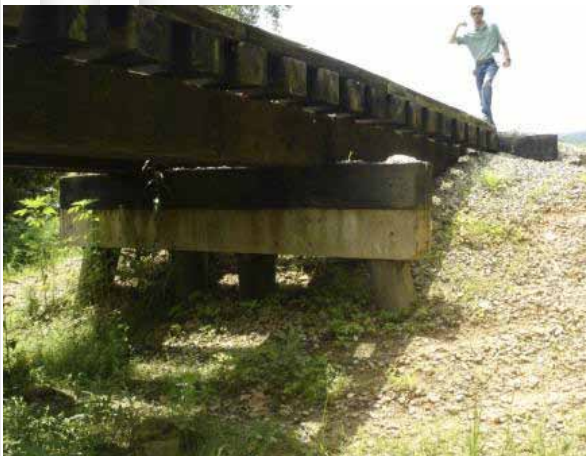
North Back Wall and Bent
