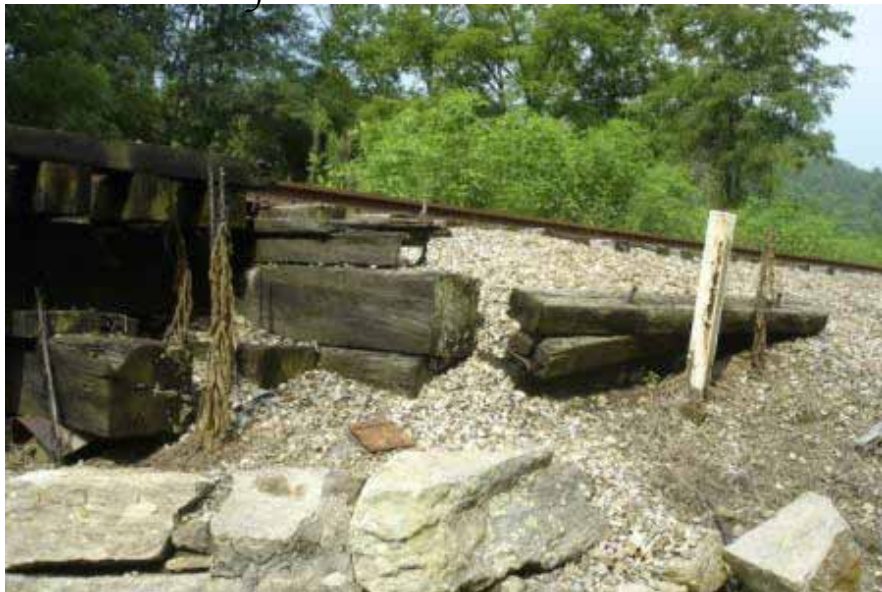
North Back Wall Undermining
