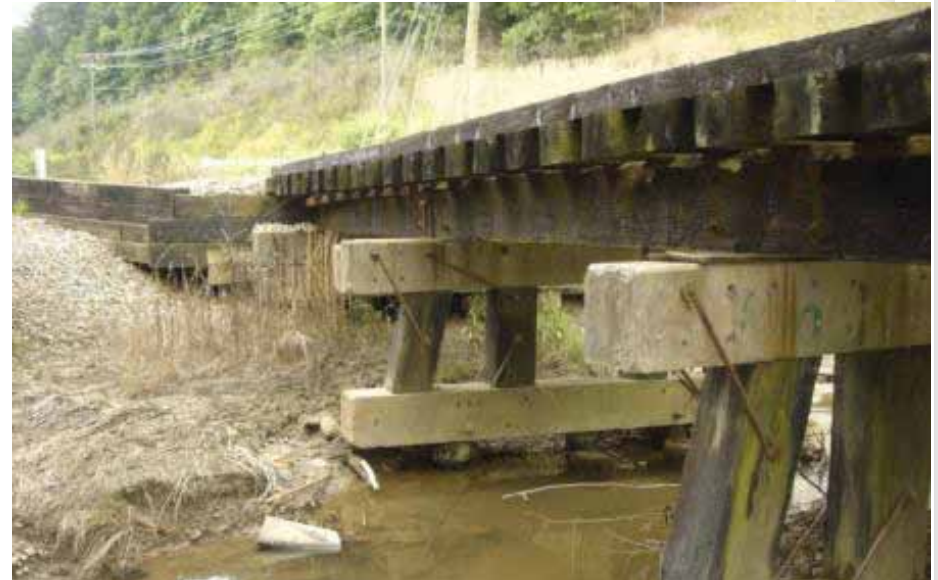
South Substructure View
