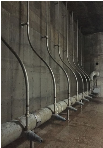
Figure 2. Interior of new ThermAer reactor with Jet Aeration Header, Blacksburg, VA
