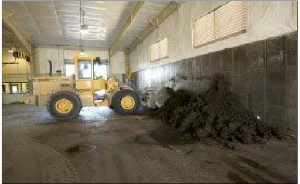
Photo 2 - Front End Loader Mixing Input Feedstocks
