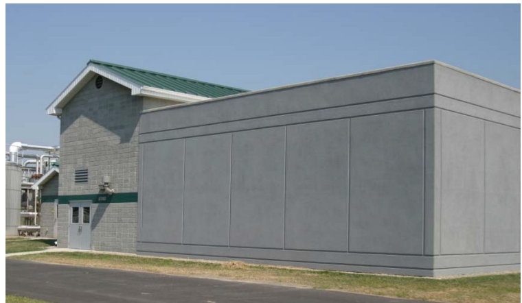
Figure 1. New Construction of ThermAer Tank System, Franklin, IN
